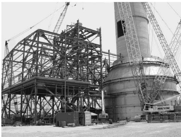
FGD Structure - August 2009
