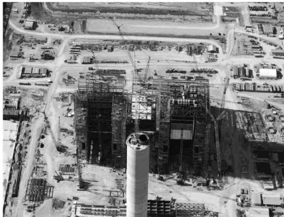
Boiler Erection, Rear View - August 2009
