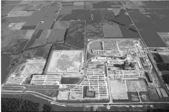
Aerial View, Late August 2009
